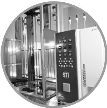
Clad Soaking System
